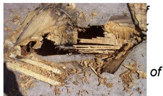
thorough inspection can usually find any soft spots under the coating that indicate weak rotted plywood/OSB board. A good estimate will include allowances for Dry-Rotted substrate.
