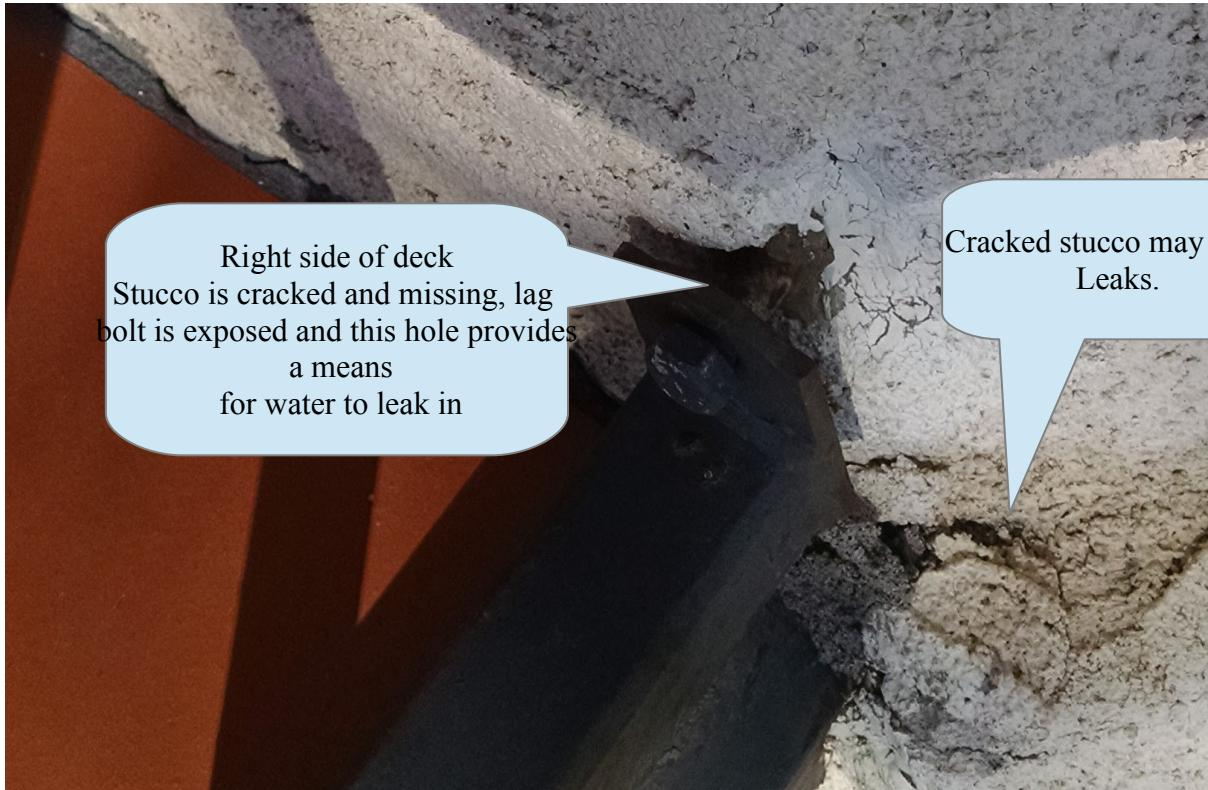
As noted above, the edge termination of this deck is highly unusual and not in keeping with standard industry design. Waterproofing/tile assemblies are typically terminated to a 26 gauge drip edge flashing. In this case, the tile terminates out onto the L bar piece of the railing. In several areas there is rust and degradation on the L bar. No waterproofing was visible at any areas inspected.
